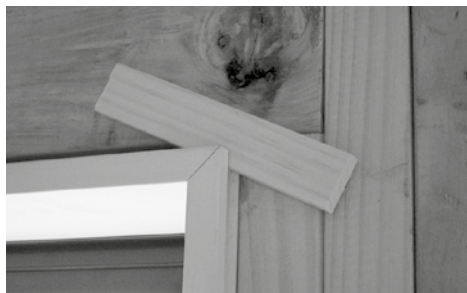
Correct installation of grooved jambs using an 11–12mm packer.
